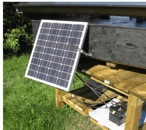
Figure 15: A solar panel and battery on a solar dryer
